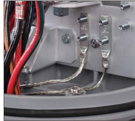
Close-up of DC trunk right side ground and drain installation.
